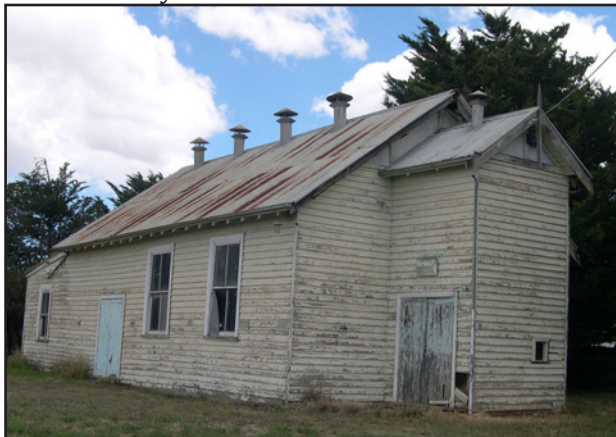
Clarkefield Hall with its bio-box out the front. This building was demolished in 2006
