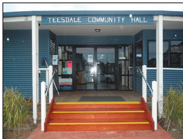
The new entrance-way to the Hall, and the defibrillator installed on the porch.
