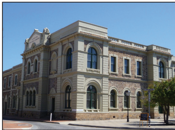
The 1876 building as it currently stands. (Photo: Joelle Hancock)
