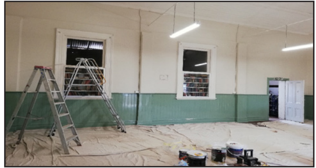
Repainting the inside of the Nagambie Mechanics' Institute. (Photo: Christine Schindler)
