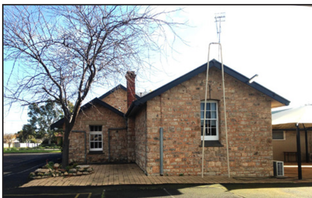
The "Bell Room" from the outside which now houses the relocated library (Photo: Peter Ralph)
