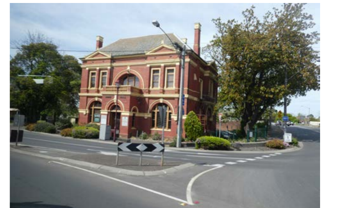
The Warragul Museum occupies the former Shire of Warragul office building.
