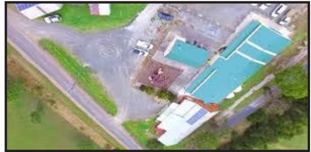
Labertouche and District Community Centre
