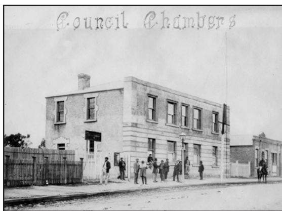
Tarnagulla Borough Council Chambers. (Photo courtesy George Swinburne)
