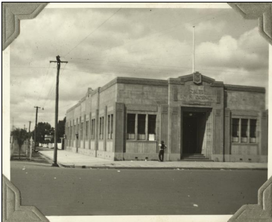
Dalby Town Council Chambers building, Dalby, ca. 1935. The School of Arts formed part of this building.
