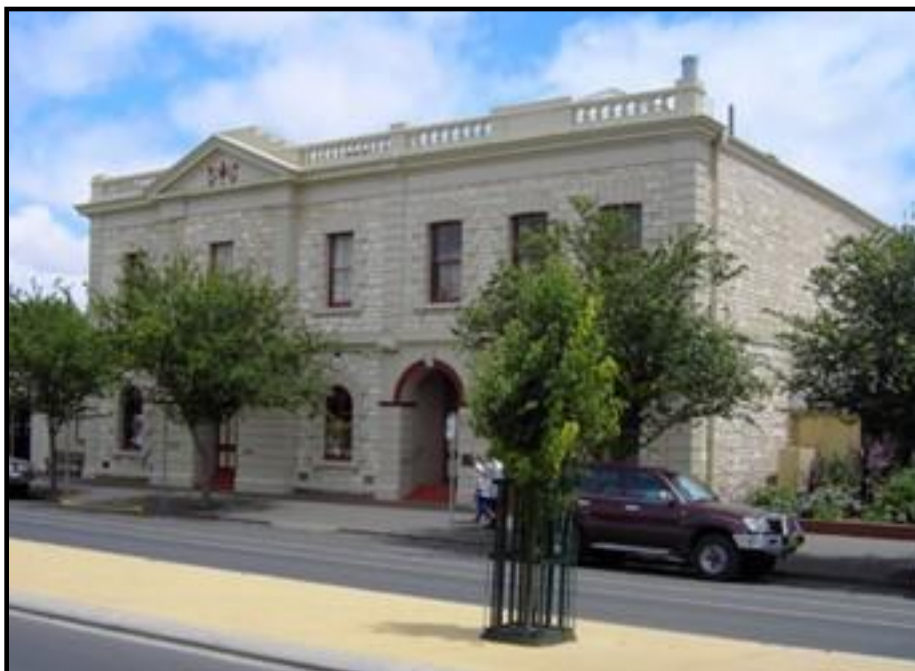
Naracoorte Institute with 1914 addition
