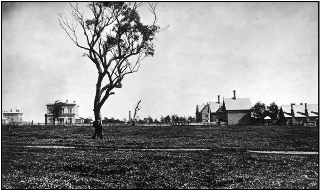
South Australia Institute building on North Terrace, 1866
