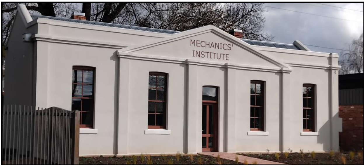
The newly restored Mansfield Mechanics' Institute
