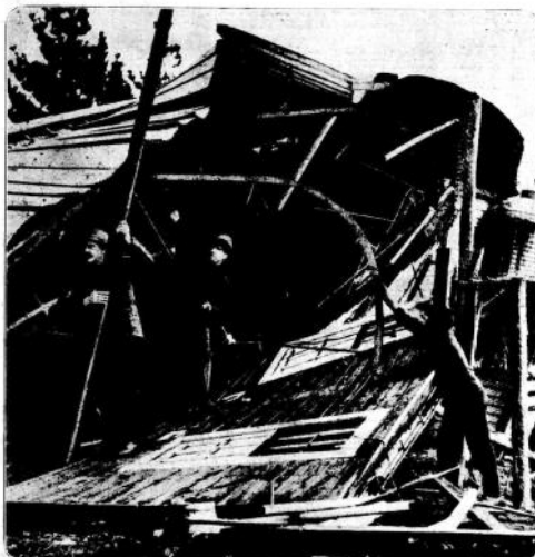
REMAINS OF THE MECHANICS' INSTITUTE IN THE TRUCK OF THE TOWN OF BUNGAREE, VIC. (Left). The picture shows the remains of the Mechanics' Institute building in the village. It has been blown down and is now a mass of twisted metal, wood and corrugated iron. The piano in the left foreground is the only one that has survived. (Right) The piano which survived the destruction of the Mechanics' Institute building. It has been blown down and is now a mass of twisted metal, wood and corrugated iron.
